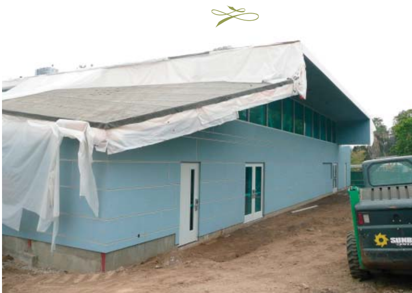
PCR Multi-purpose room construction is nearly finished
