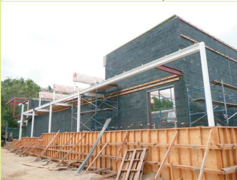
PCY multi-purpose room construction is progressing steadily
